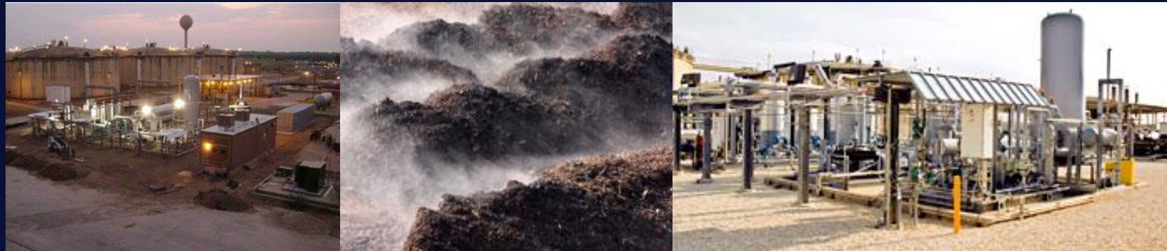
[Photo Credit: San Antonio Water System]
